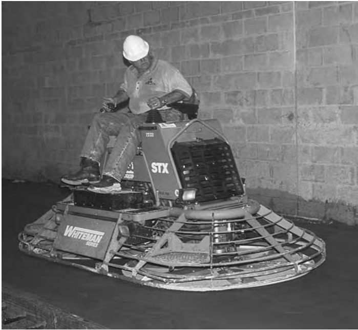
Figure 17.8 Riding trowel machine fitted with float pans
